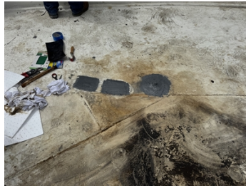
Belzona 1212 Tank patches view 2
