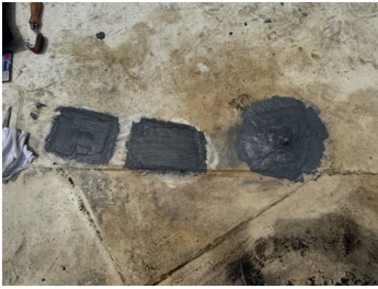
Belzona 1212 Tank patches view 1.
