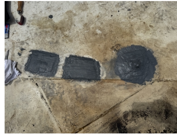
Belzona 1212 Tank patches view 3
