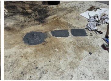
Belzona 1212 Tank patches view 4
