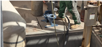
Pump pedestals being blasted
