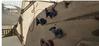
Pump pedestals first coat with Belzona 4311
