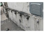
The large water tank with Showing a small, but costly leak Showing plate bonding to a live Another angle of the repair compromised liner and through toward the bottom of the tank leak using Belzona 1212 wall leak
