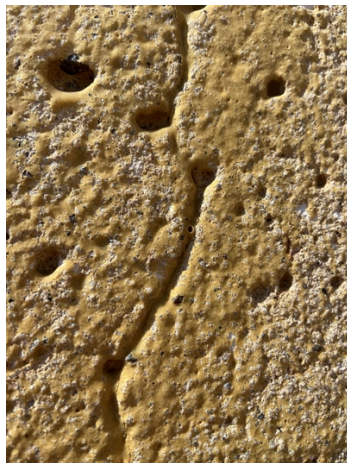
Close up photo of a defect in the sump wall.
