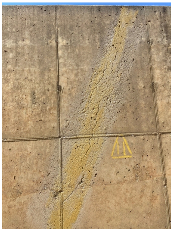
Crack in concrete along the wall of sump.
