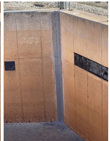
Floor to wall joint crack repair in grey, and existing previous Belzona crack repair in black still in good condition.
