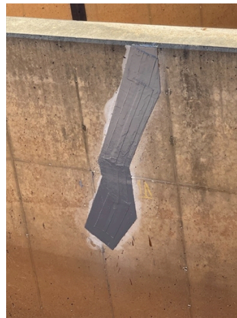
Belzona 5815 and 9371 crack repair on the application area.
