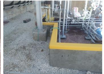
About 1.5 years after install we completed a visual inspection of the coating and it was still in good condition.
