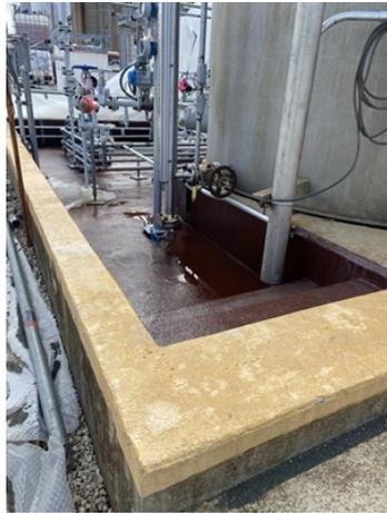
Belzona 4311 applied into containment
