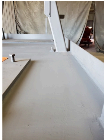
Belzona 1121 applied and smoothed over pitting
