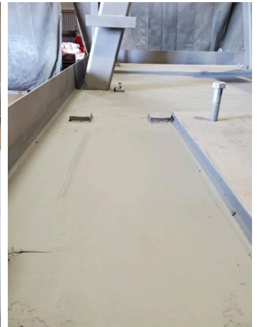
Belzona 1121 applied and smoothed over pitting
