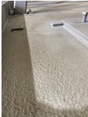
Skid after abrasive blasting
