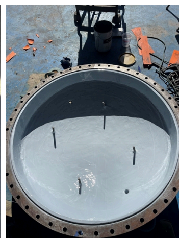
Final result with two coat system of Belzona 1321
