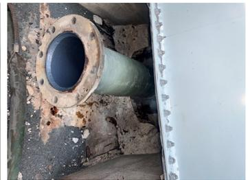
Before image of the sump with existing polyurea liner on it. Internal view.
