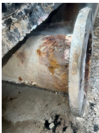
Before image of the discharge pipe coming off of the sump. External view.
