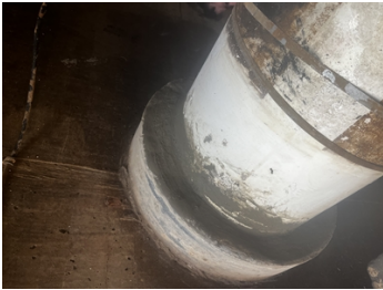
Leaking pipe penetration
