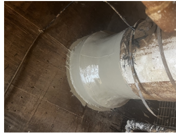
The finished product using Belzona 5815 with 9311 reinforcement
