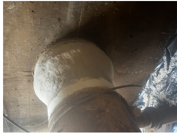
Building up around pipe from concrete with Belzona 4141
