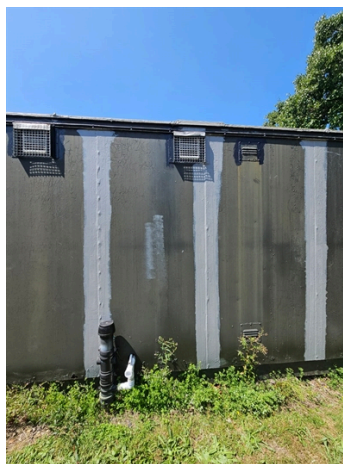
Belzona repairs carried out by one of the client's contractors
