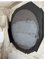
Rebuilding damaged areas using Belzona 1111 (Super Metal) to restore metal loss and ensure structural integrity.
