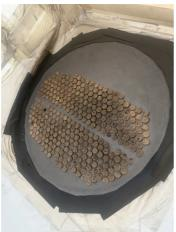
Surface after abrasive blasting, showing a clean and profiled tube sheet ready for application. Tubes protected using corks.
