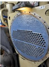
Completed application of Belzona 1321 in two coats with plugs removed, revealing a smooth and fully protected tube sheet surface.
