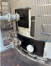
Insulation removed and can see Abrasive blast completed per the pitting / external corrosion SSPC-SP10 on the nozzles
