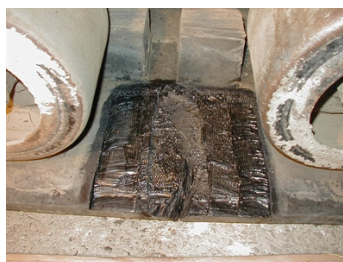
A grinder was used to prepare the substrate. Belzona 2911 (QD Conditioner) was applied to the prepared area.
