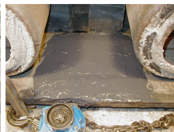
The area was built up with Belzona 2211 (MP Hi-Build Elastomer).
