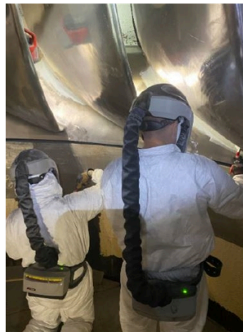
Application of 1st coat of Belzona 1341
