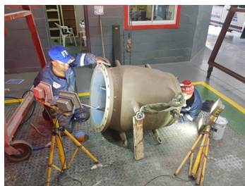
First coat of Belzona 1321 being applied
