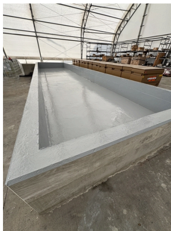
Containment - Final/Second Coat with Belzona 5811 (Grey)
