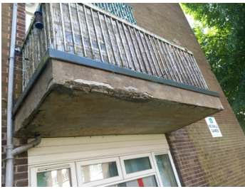
Badly spalled concrete to under-ledge of balcony
