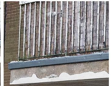
A further angle, showing 1 of 20 successful concrete repairs, some 18 months later
