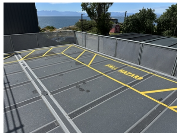
High visibility markings identifying fall hazard
