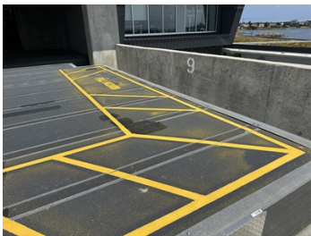
Clean lines, 3 coats total were applied
