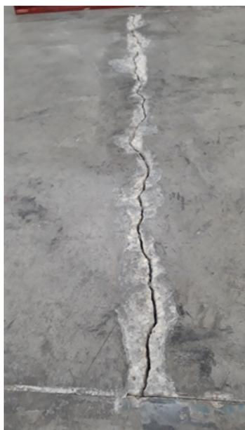
Cracks, showing prep to sides and solid surrounding substrate
