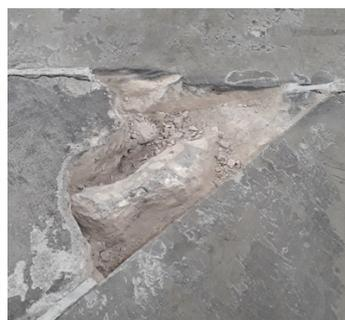
Further damage to adjacent slabs, causing issues for FLT Traffic
