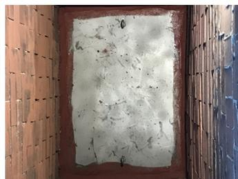
A steel plate was employed to seal over the damaged floor, this was grouted in with Belzona 4311 CR1 prior to encapsulating the whole sump
