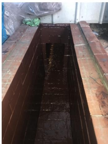
The trough completely lined and sealed
