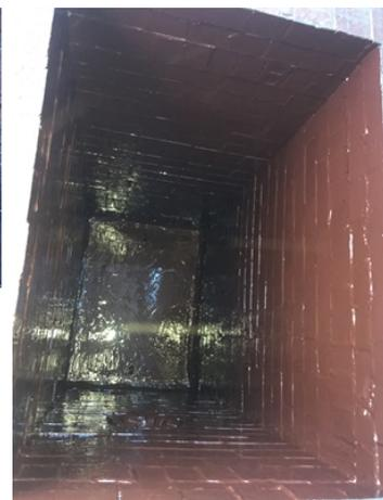
The sump with a new base plate, completely encapsulated
