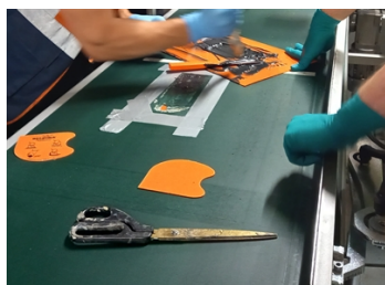
Area taped off and wetted out, Belzona 2311 applied following
