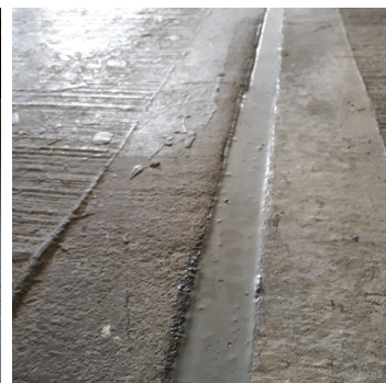
Completed works showing the Belzona 4521 still in it's intended location
