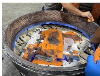
Applying Belzona 9811 alumina tiles
