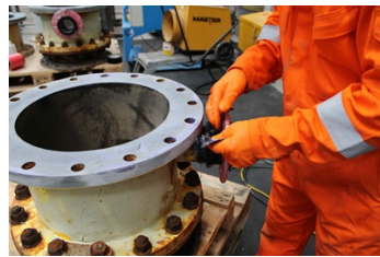
Belzona 7311 is applied and Belzona Superwrap II is applied to add strength and integrity
