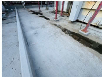
Belzona 5815 pictured (14 months in service)
