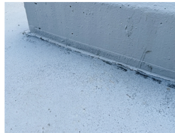
Belzona 5815 (14 months in service) used with 9371 composite reinforcement tape. This was applied to all seams and perimeters where the walls met the floor.
