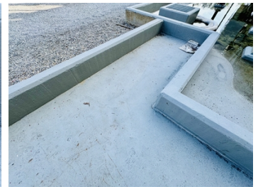
Belzona 5815 (14 months in service)
