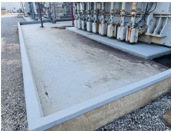
Belzona 5815 pictured (14 months in service)
