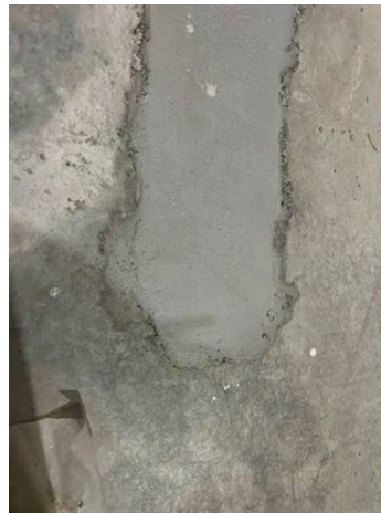
Repaired crack area on side of pump base using Belzona 4111
