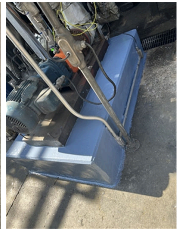
Completed repair and coating of concrete pump base using Belzona 4111 and Belzona 5821
