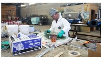
Contractor initial mixing of Belzona 1813.
