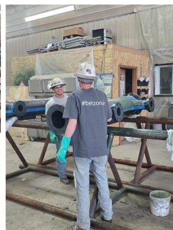
Belzona 1813 applied to fiberglass headers.
