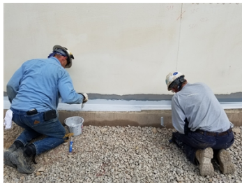
Belzona 3131 (WG Membrane) being brush applied with 9351 reinforcing sheet.
