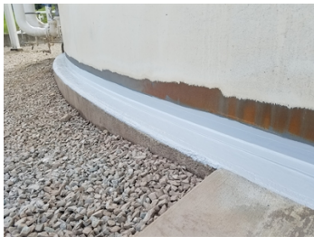
Finished application. Customer will go back with their tank paint to touch up areas that were grit blasted but not coated.
