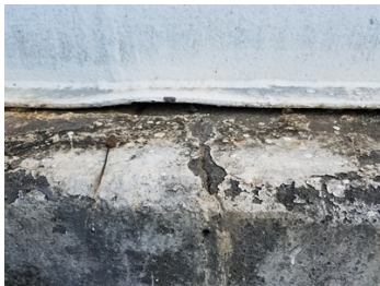
An example of the condition of the chime angle prior to any work starting.
