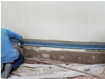
Belzona 3931 (WG Membrane Conditioner) being brush applied.
