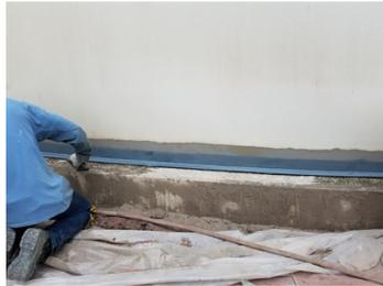
Belzona 3931 (WG Membrane Conditioner) being brush applied.
