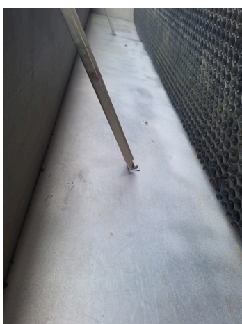
Surface preparation prior to Belzona systems being applied
